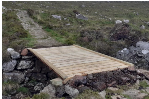
Completed bridge on Abhainn an t-Sratha.
