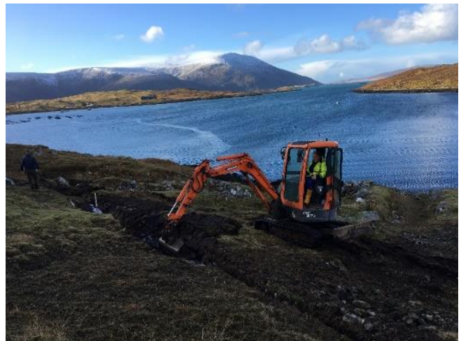
Whaling Station Drainage
